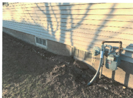
Storm windows to be removed and blocked up (2 windows are under the front deck)
