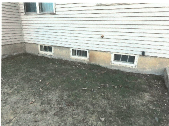
Storm windows to be removed and blocked up (2 windows are under the front deck)
