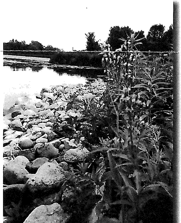
Shoreline stabilized with riprap and enhanced with a vegetative buffer.
