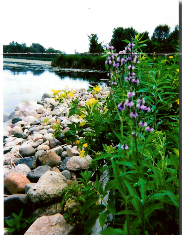
Shoreline stabilized with riprap and enhanced with a vegetative buffer.
