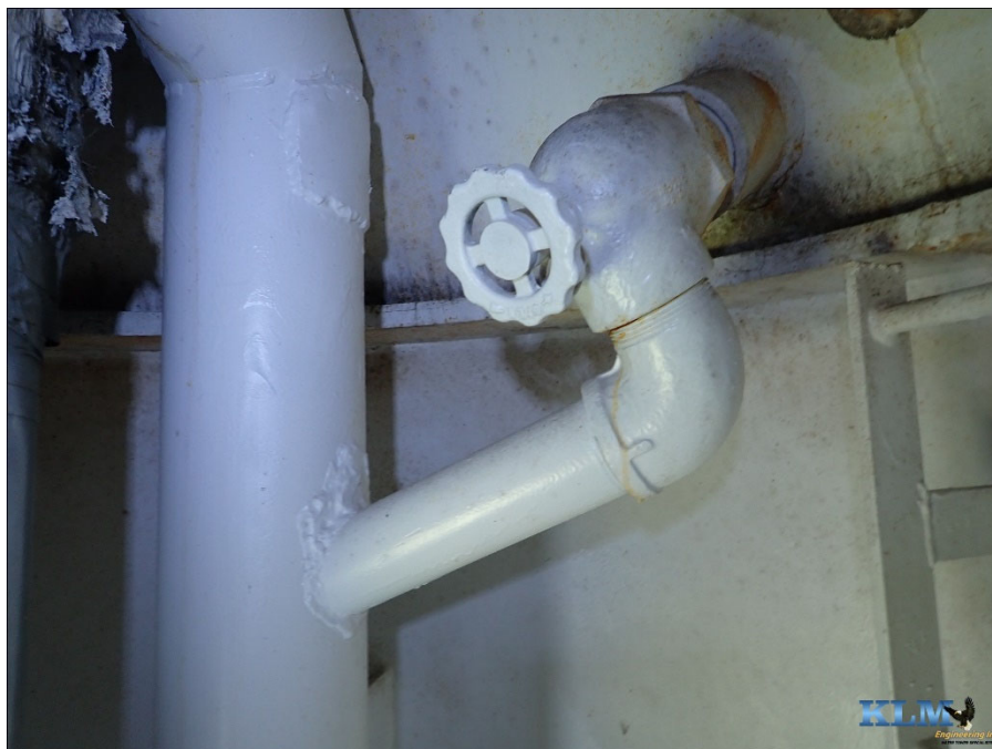
Photo No. 27 Bowl drain cleanout
