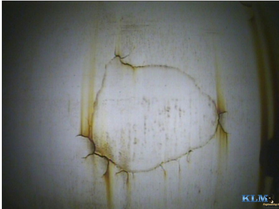
Photo No. 23 Coating failures and corrosion on shell, Note; indication of poor surface preparation during repairs
