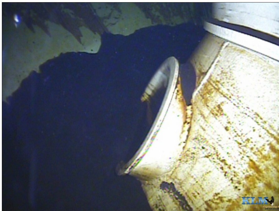
Photo No. 12 Sediment accumulation in bowl
