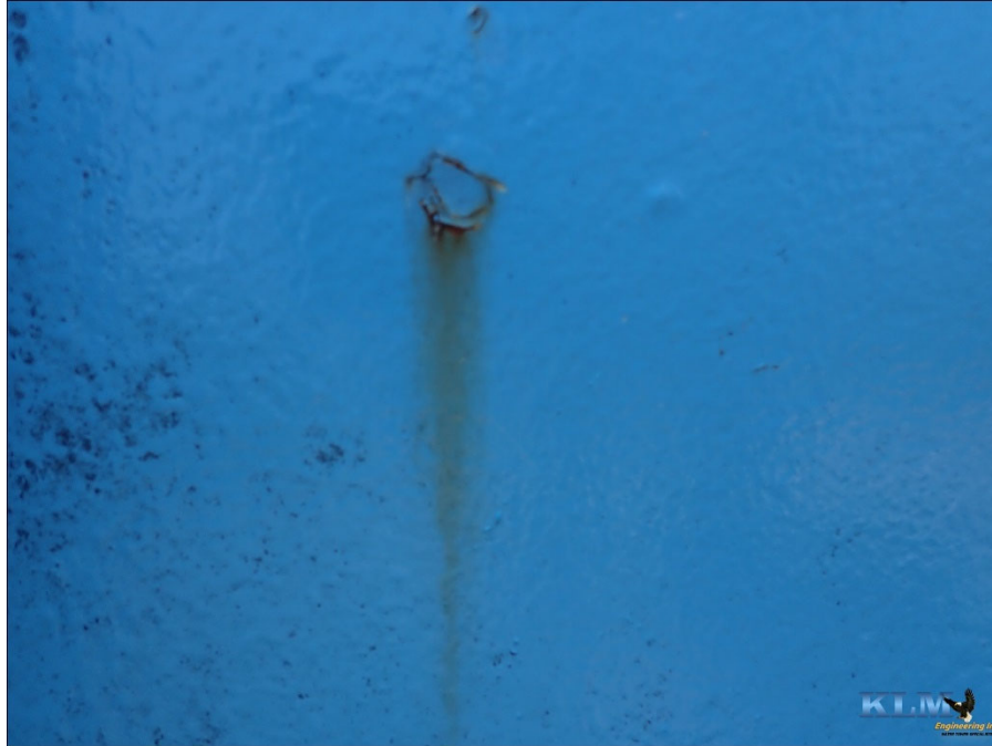
Photo No. 47 Isolated corrosion on base cone
