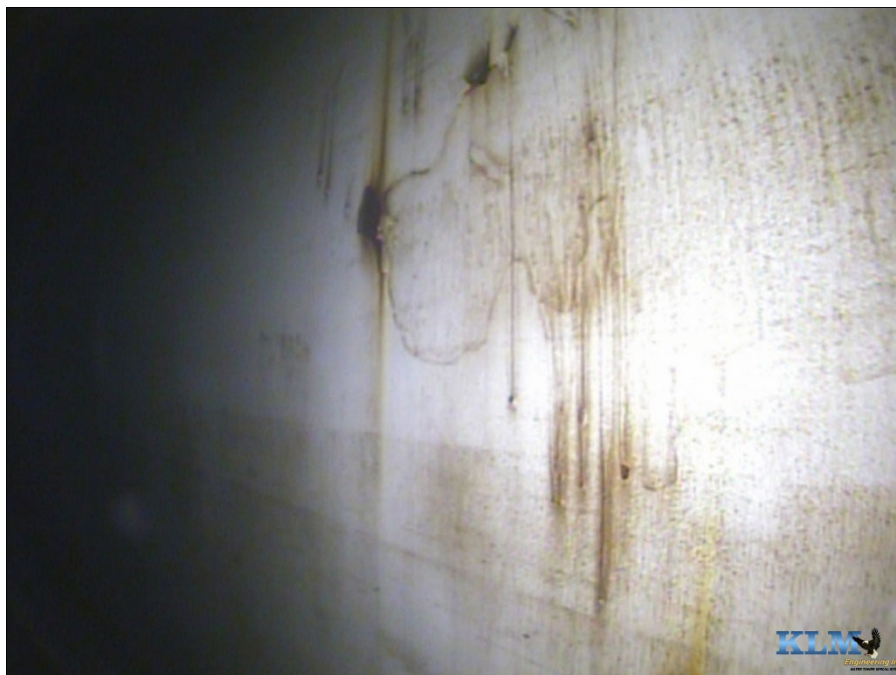
Photo No. 22 Coating failures and corrosion on shell, Note; indication of poor surface preparation during repairs
