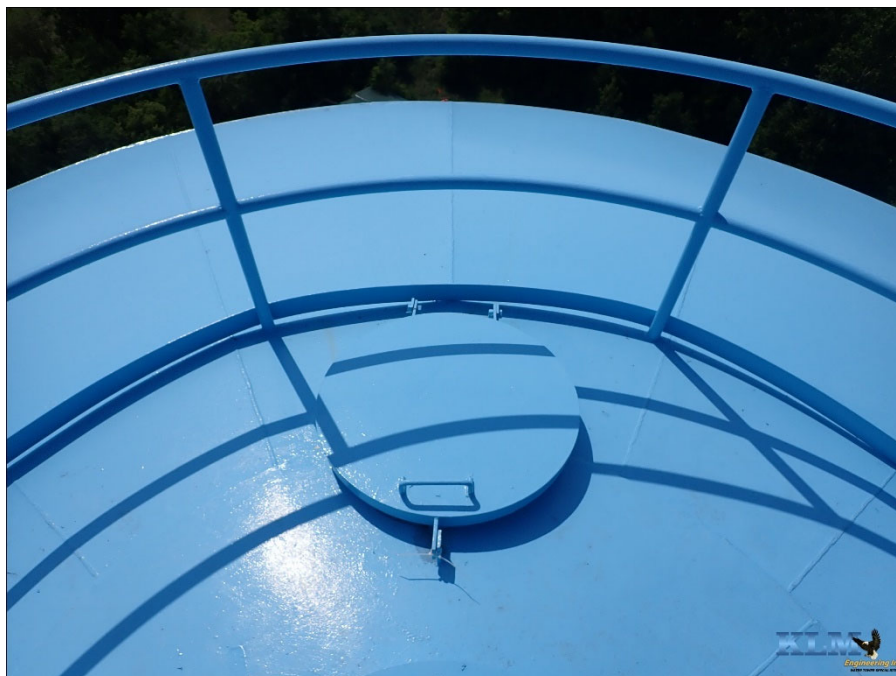
Photo No. 39 Access manway and roof conditions
