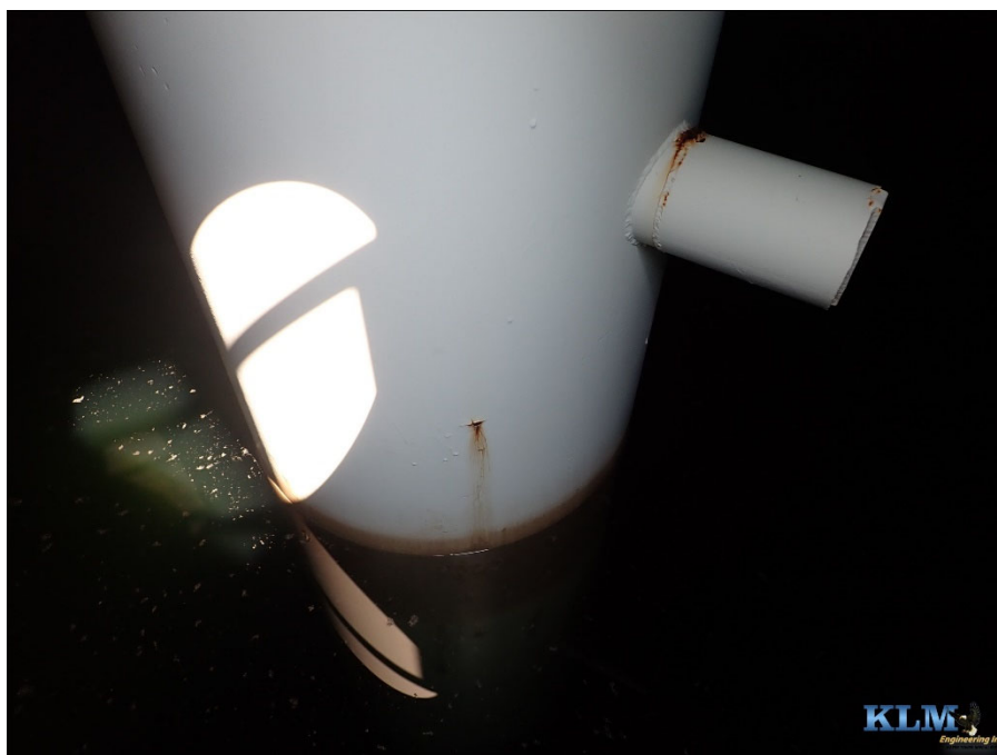
Photo No. 8 Drywell tube and overflow
