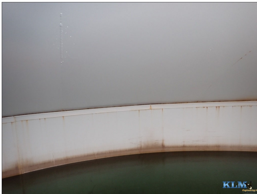
Photo No. 7 Roof condition and connection to shell
