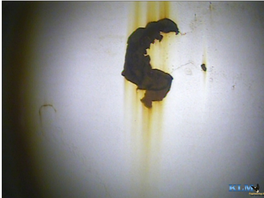
Photo No. 21 Coating failures and corrosion on shell, Note; indication of poor surface preparation during repairs
