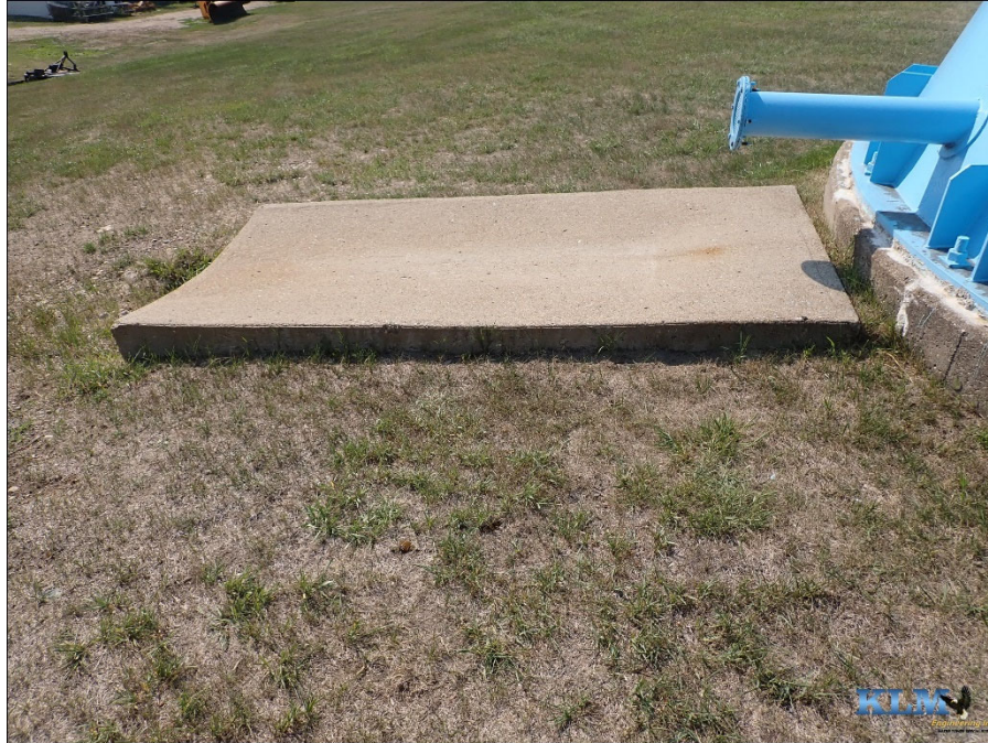
Photo No. 49 Overflow and splash pad
