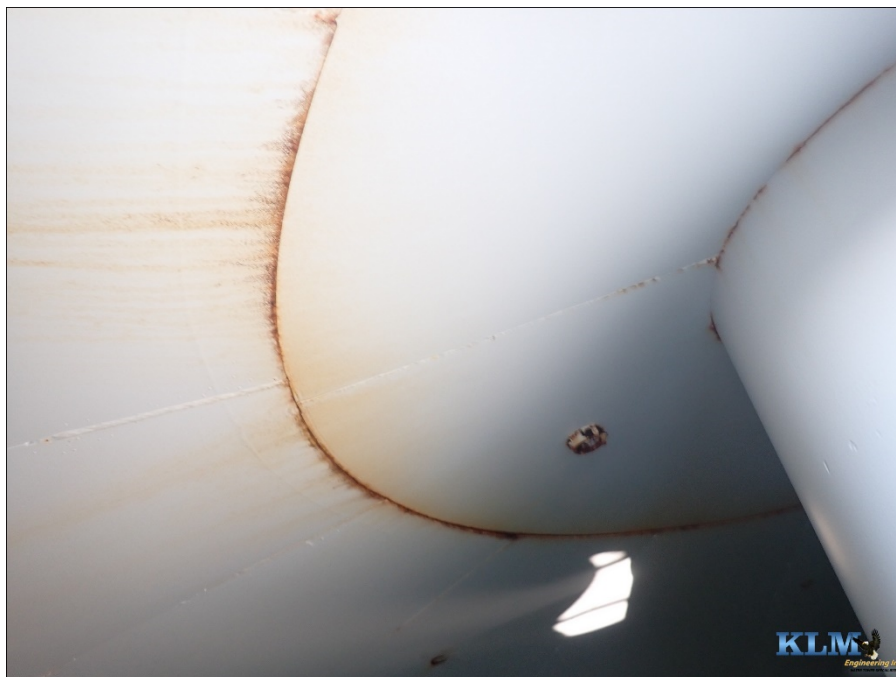
Photo No. 2 Dollar plate to drywell tube and roof plate, Note; rigging coupling
