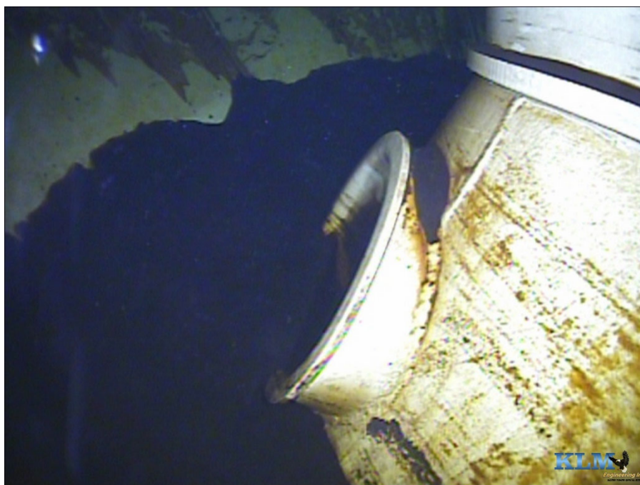
Photo No. 12 Sediment accumulation in bowl
