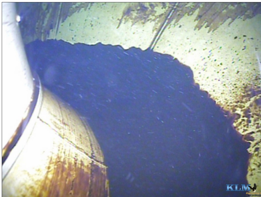
Photo No. 11 Sediment accumulation in bowl
