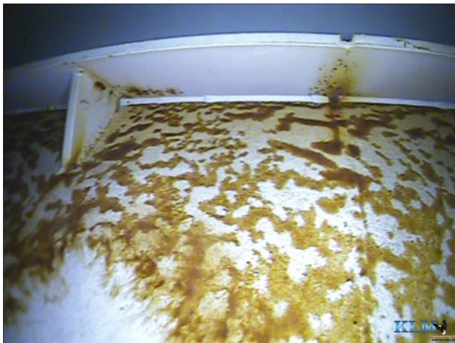
Photo No. 17 Leveling ring at bowl to shell connection
