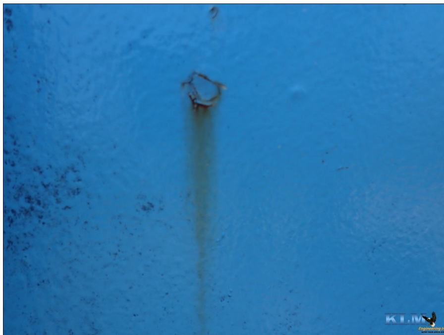
Photo No. 47 Isolated corrosion on base cone
