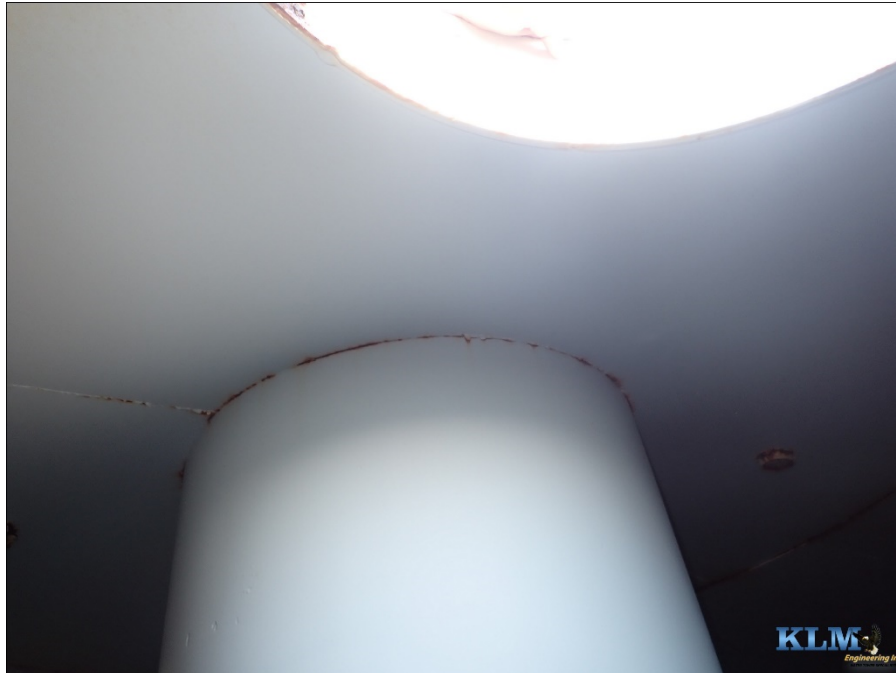
Photo No. 3 Drywell tube to roof connection
