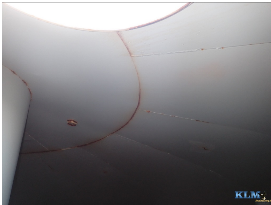
Photo No. 4 Dollar plate to drywell tube and roof plate, Note; rigging coupling
