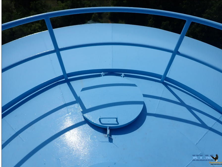
Photo No. 39 Access manway and roof conditions
