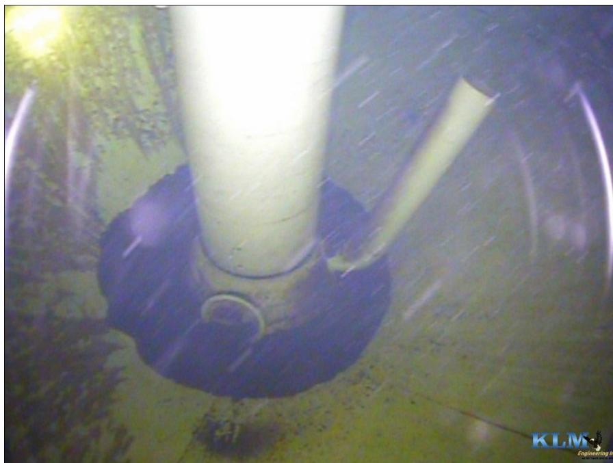
Photo No. 10 Drywell tube and bowl, Note; fill pipe and manway
