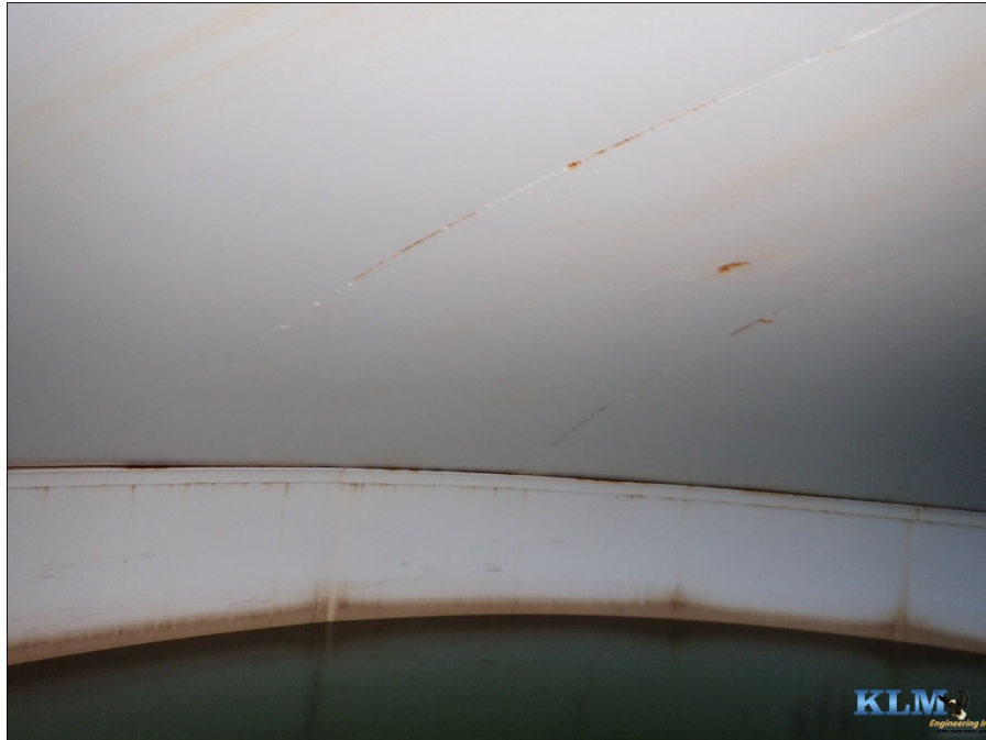
Photo No. 5 Roof condition and connection to shell
