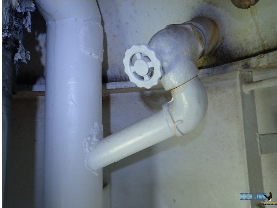
Photo No. 27 Bowl drain cleanout
