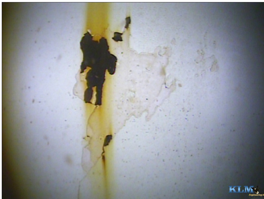
Photo No. 20 Coating failures and corrosion on shell, Note; indication of poor surface preparation during repairs
