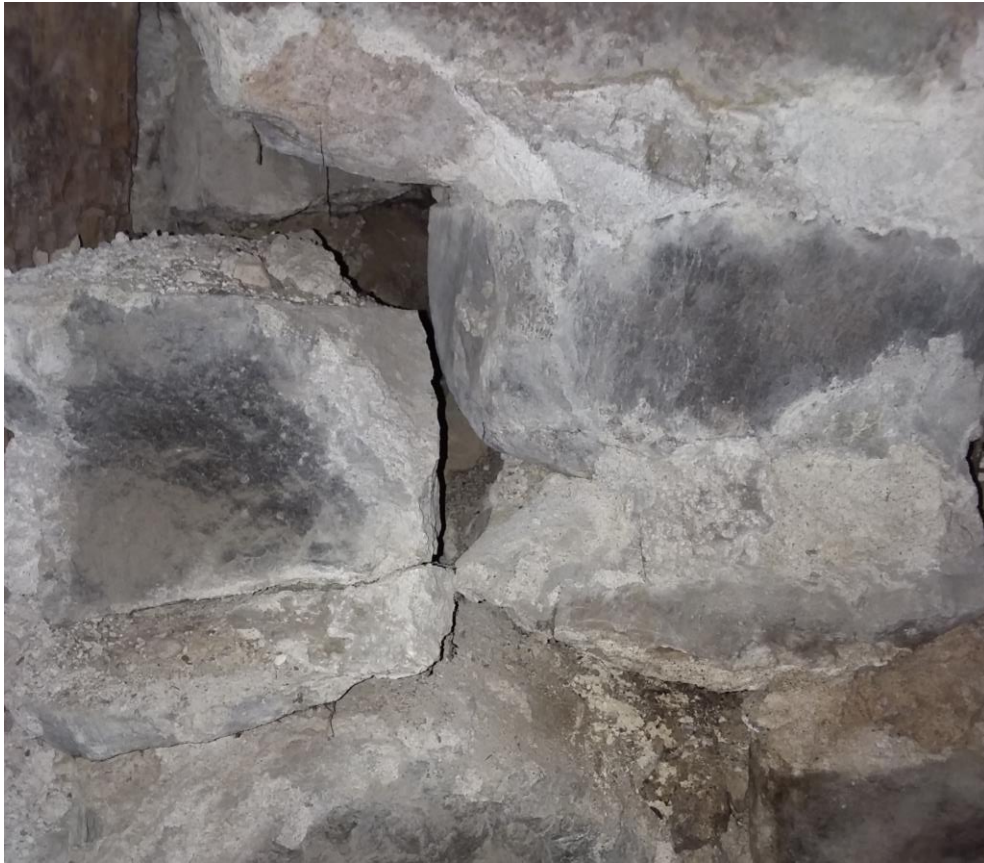
Photo #11 – Large voids in south foundation wall
