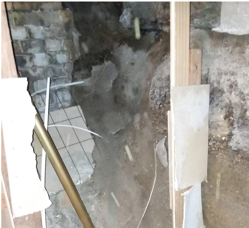
Photo #5 – Foundation wall failure at northwest corner
