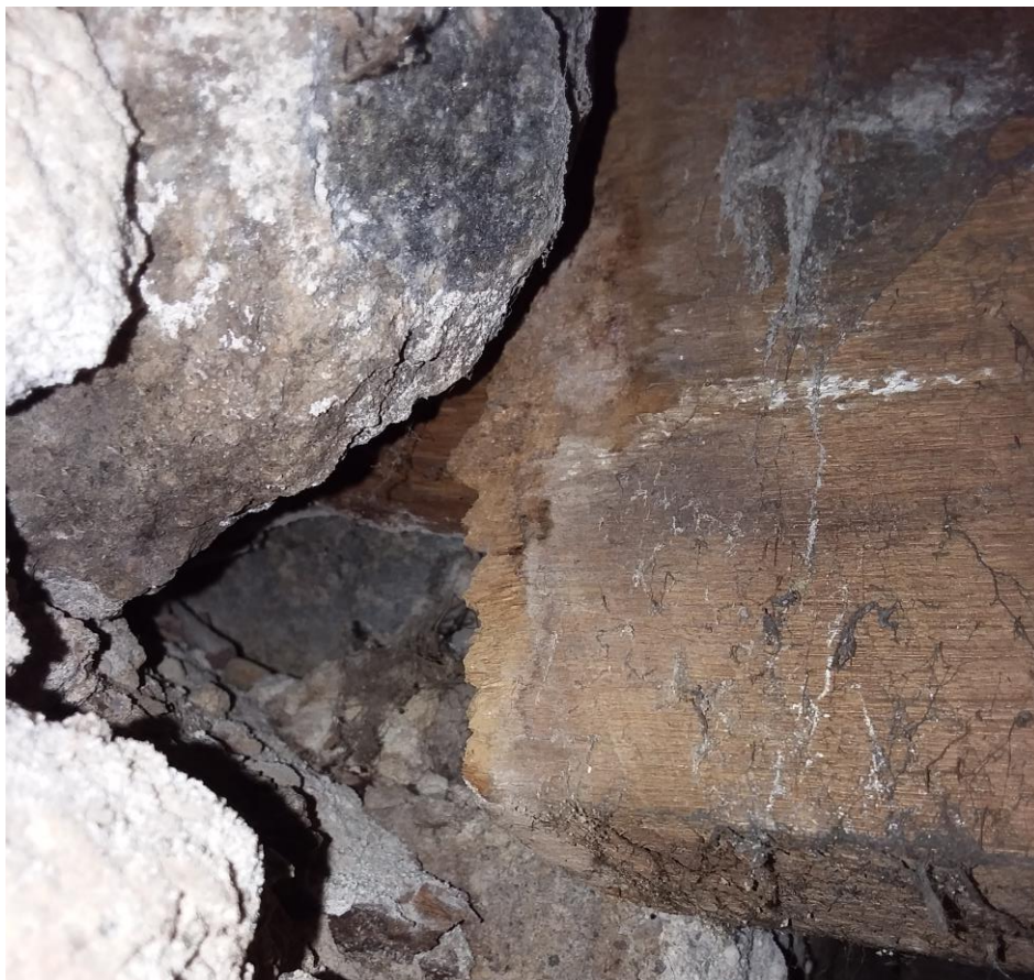
Photo #17 – Joist deterioration at east wall
