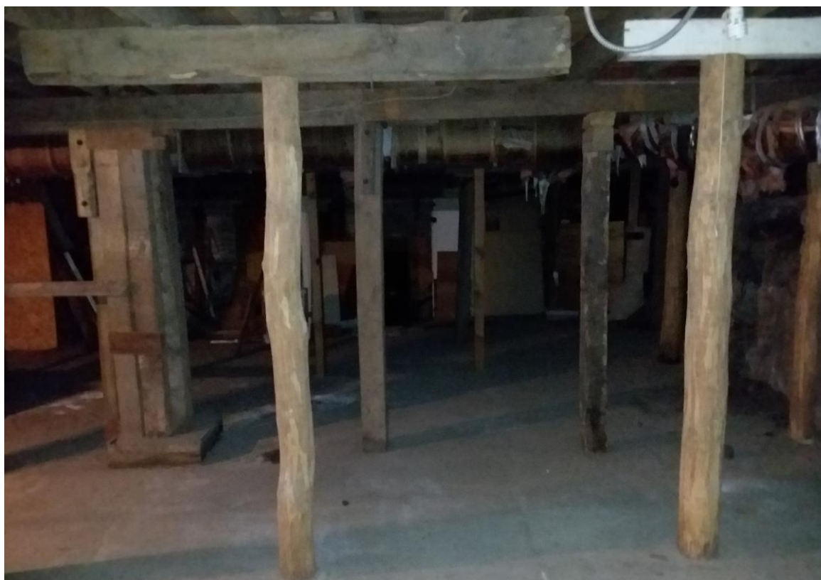
Photo #14 – Additional beams and columns supporting floor system
