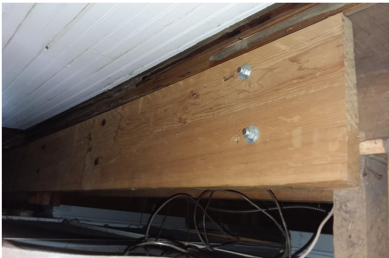
Photo #20 – Wood beam reinforcement
