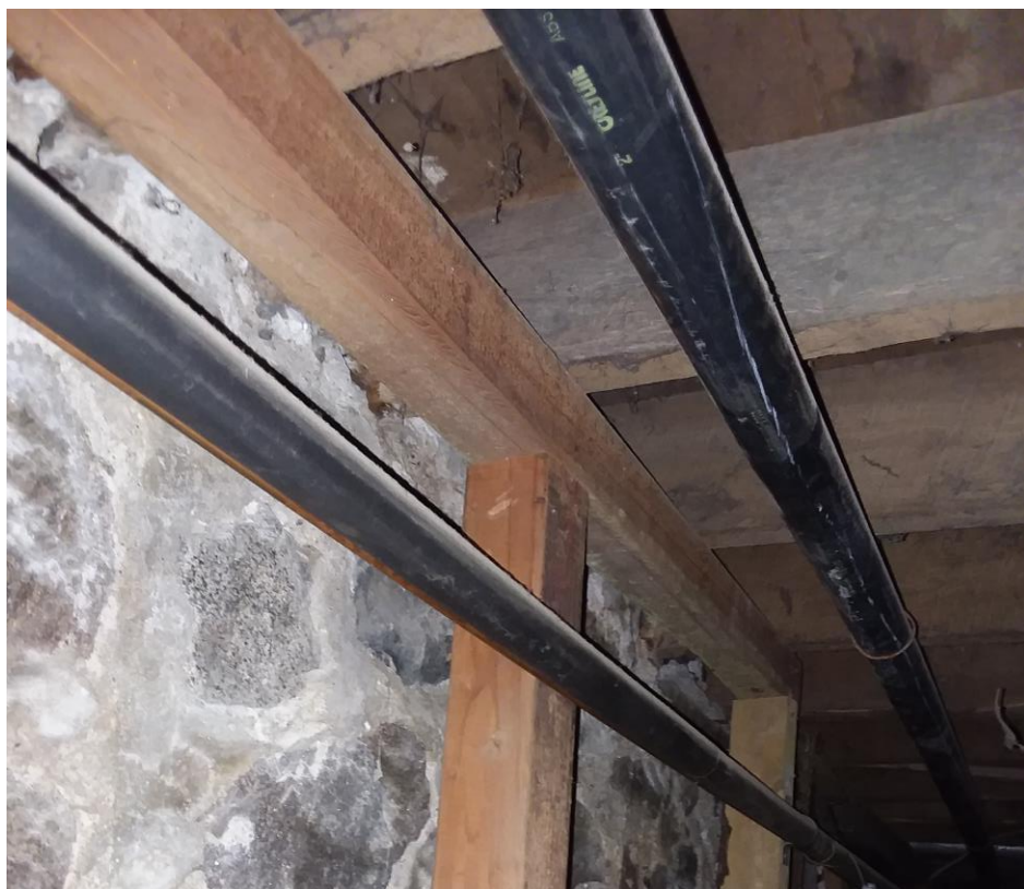
Photo #18 – Beam and column below joists at east wall
