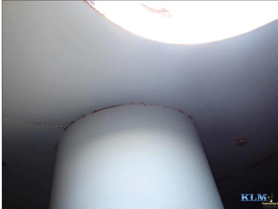
Photo No. 3 Drywell tube to roof connection
