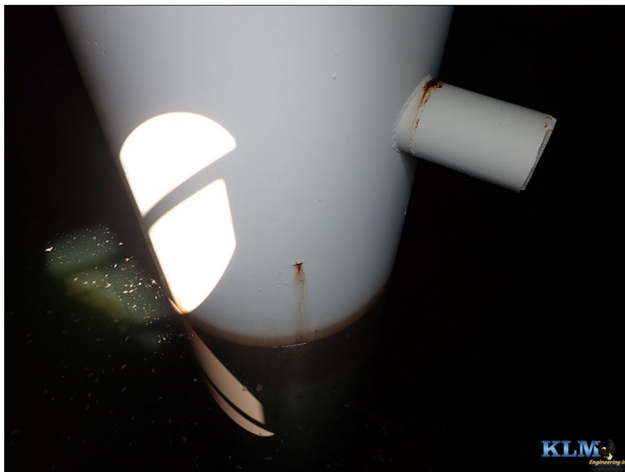
Photo No. 8 Drywell tube and overflow
