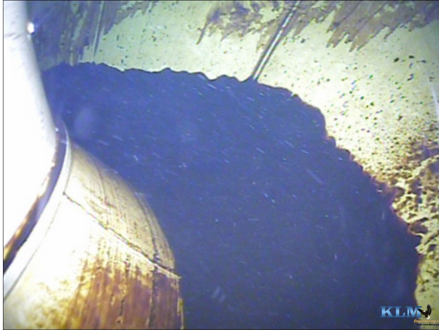
Photo No. 11 Sediment accumulation in bowl
