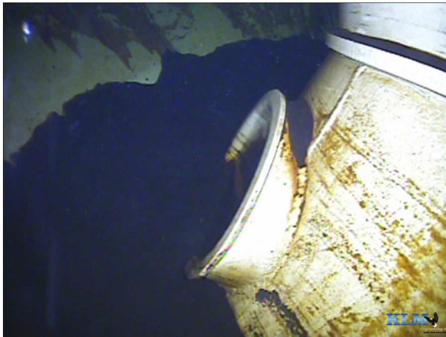
Photo No. 12 Sediment accumulation in bowl
