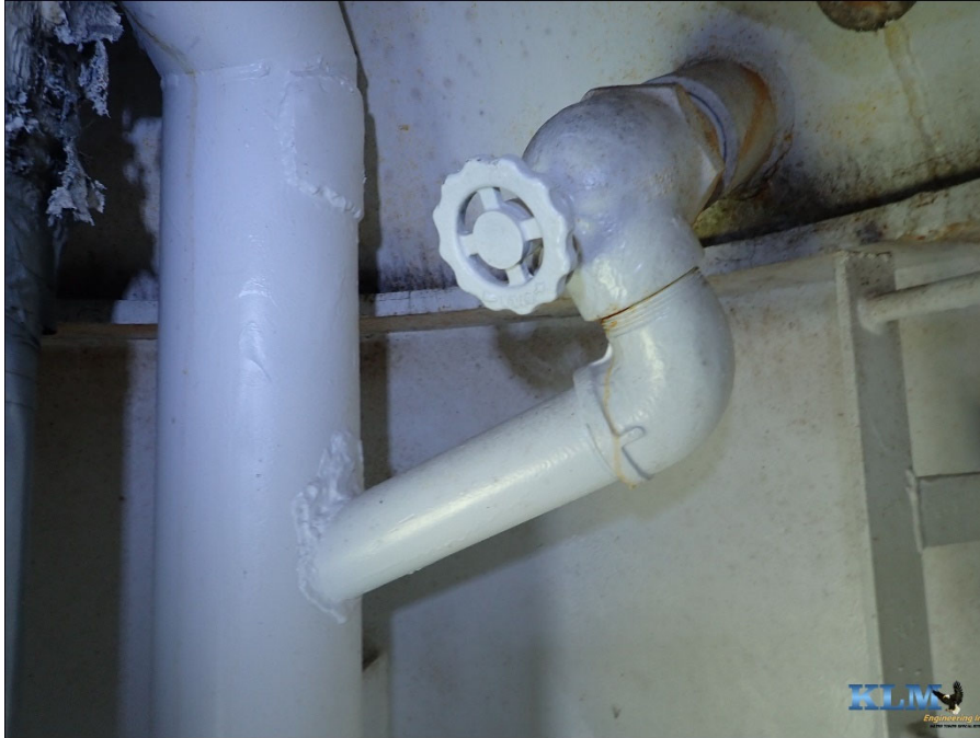
Photo No. 27 Bowl drain cleanout
