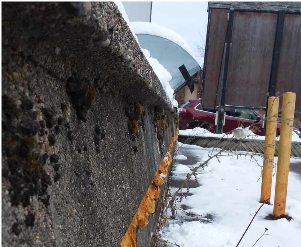
Photo #12 – Distressed masonry wall on east side of building
