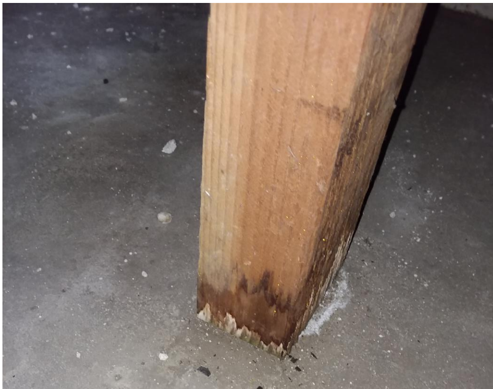
Photo #15 – Moisture at bottom of column
