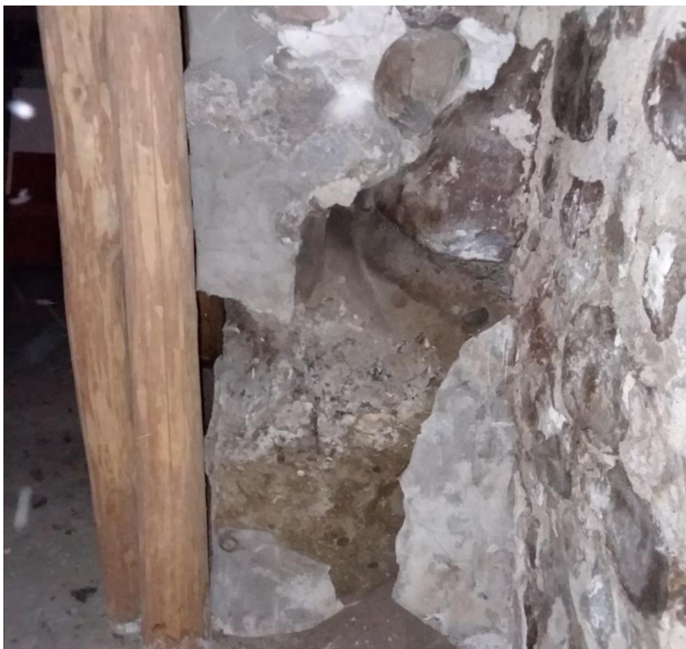
Photo #10 – Pier deterioration on north wall
