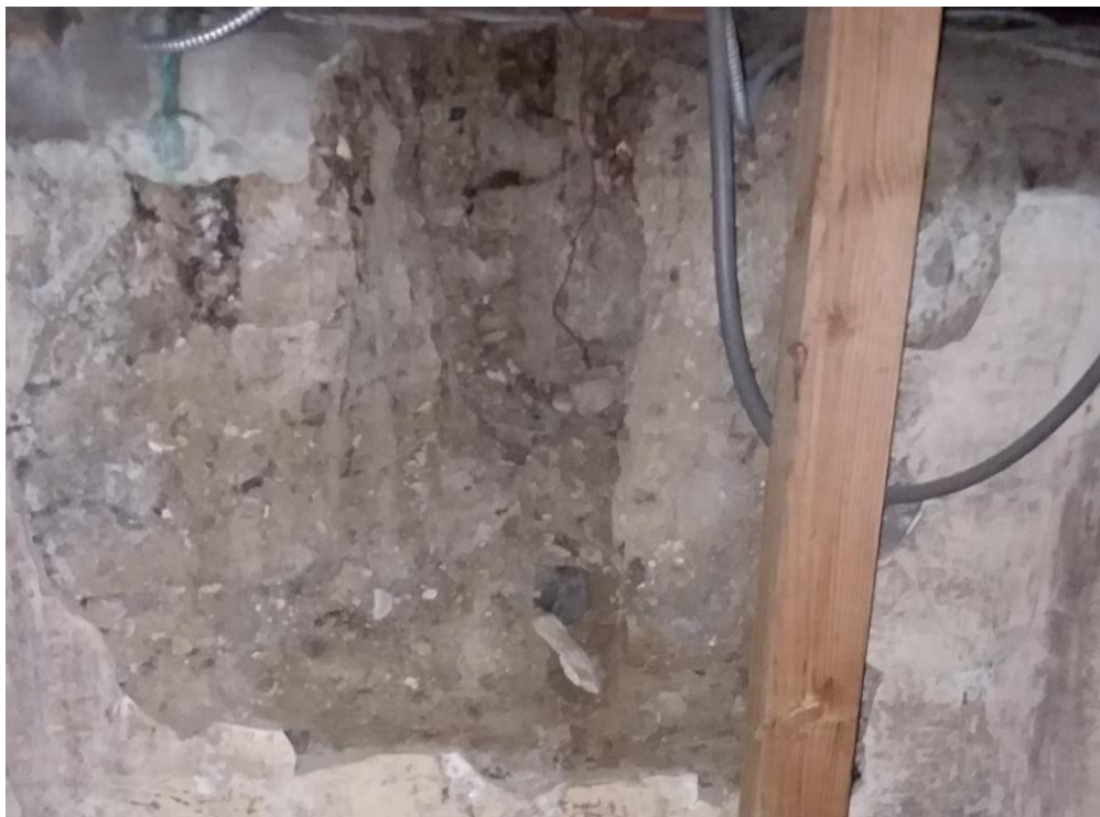
Photo #9 – Foundation failure on south end of crawl space
