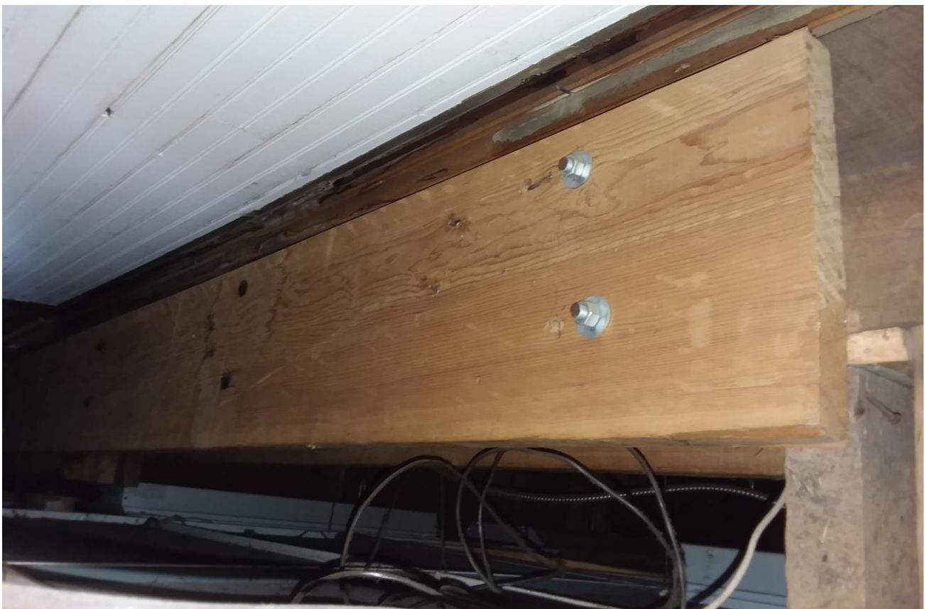
Photo #20 – Wood beam reinforcement
