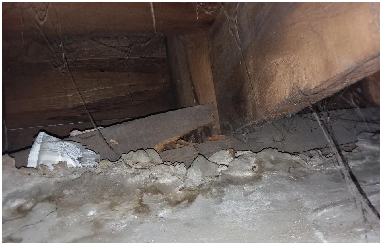
Photo #16 – Rotted plate below floor joists on west wall
