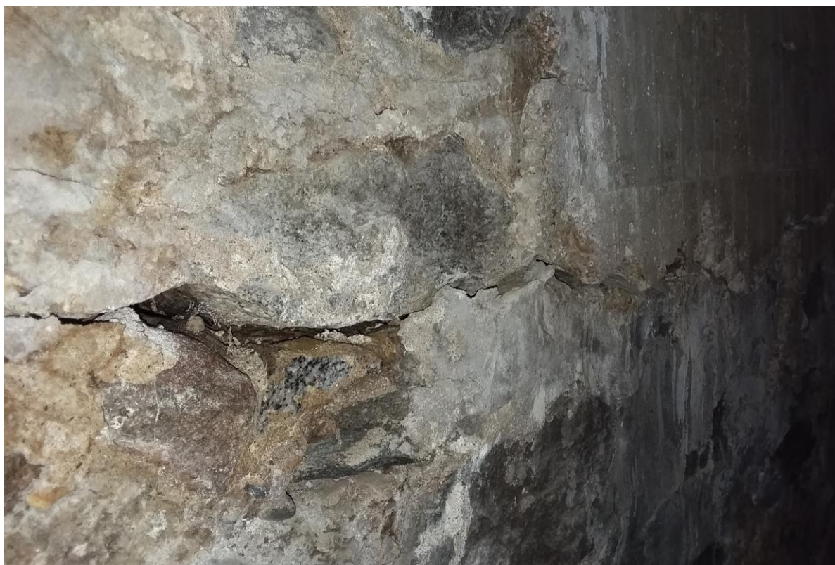
Photo #6 – Horizontal crack at north end of east wall
