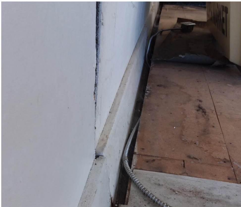
Photo #13 – Gap between east wall and floor sheathing
